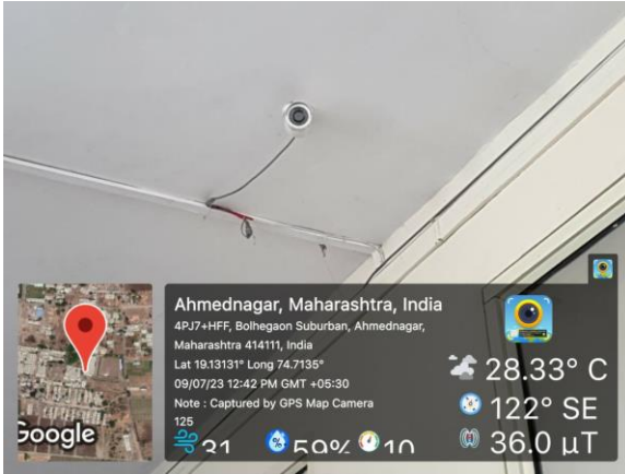
Camera 2 First Floor Porch
