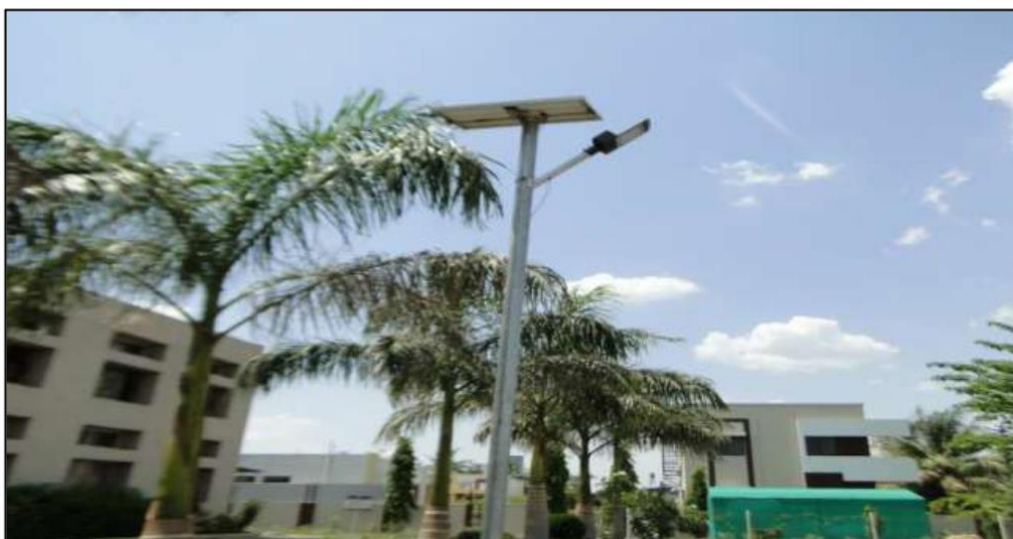
Installation of Solar Lamp in College Campus
