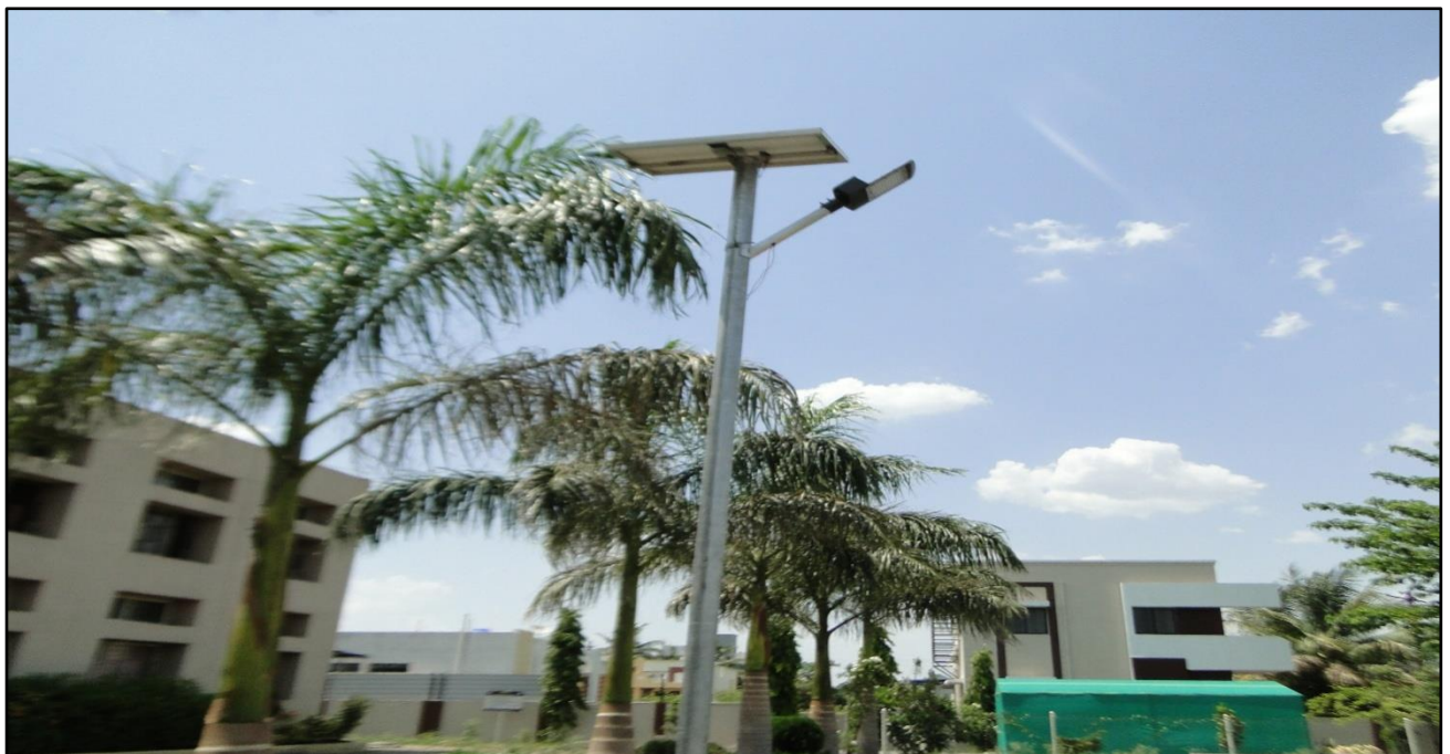
Installation of Solar Lamp in College Campus
