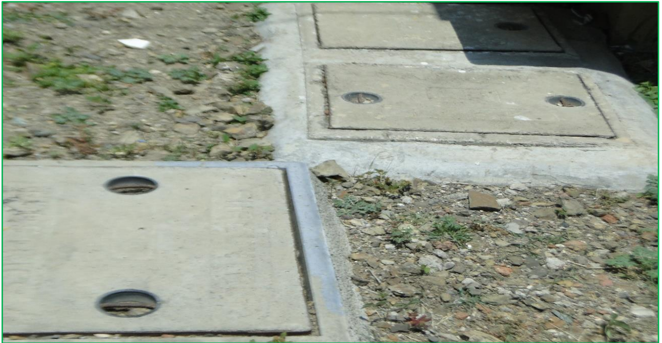
Rainwater Deposited Pit
