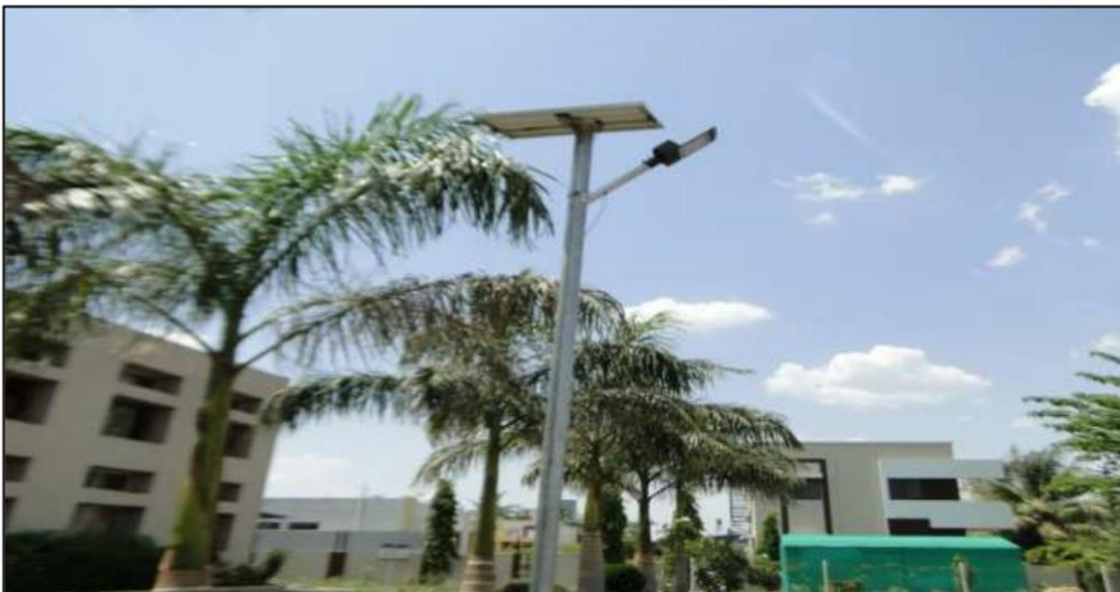
Installation of Solar Lamp in College Campus
